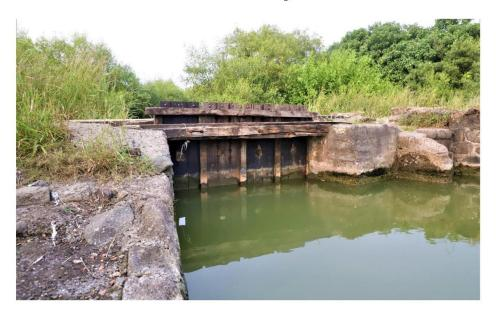
**Image 2:** Wooden sluice gate on the water channel at TSC.
