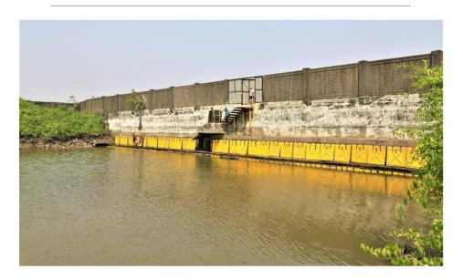
**Image 1:** Tide gate on the creek at Panje Wetland. Image shows upper 35 flip valves while lower 35 valves are submerged. Currently these flaps are open allowing tidal water to flood the wetland. The closer of these flaps will kill the entire wetland
