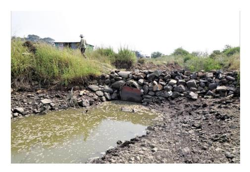
Image 3: Single concrete pipe culvert with a door at Panje Wetland.
